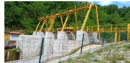
Stenjevec SmallHydro (902 kW, Francis)
